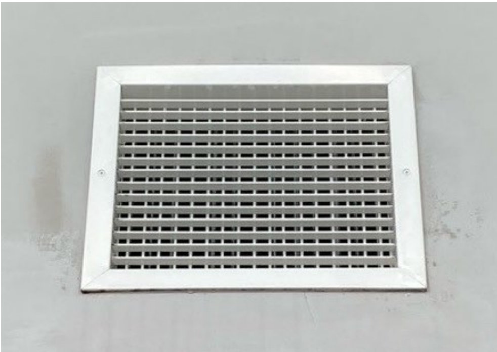
Moisture around an air register
