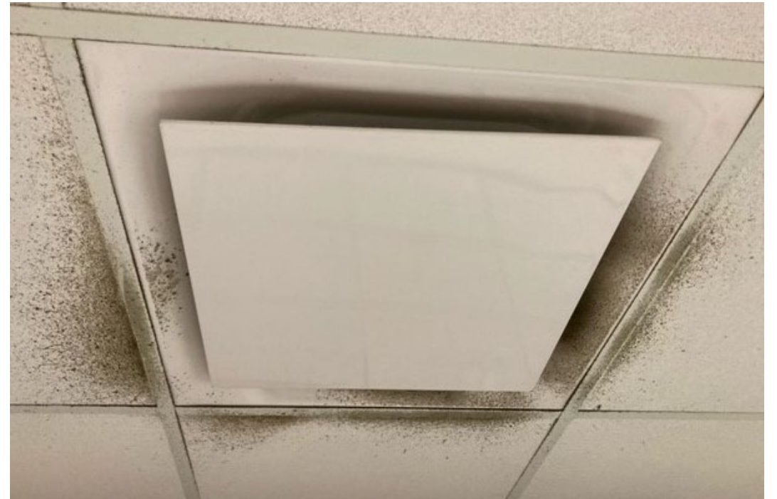
Moisture and dust around an air diffuser
