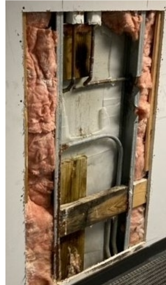
Mold inside a wall caused by a water leak
